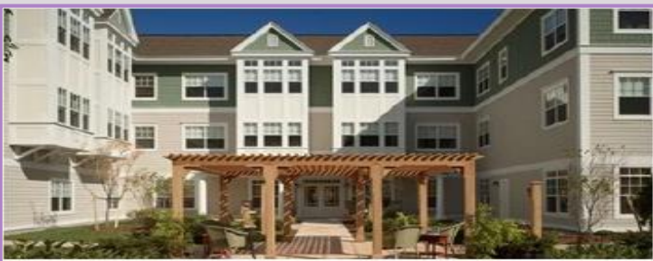
A larger facility may be able to offer more services and amenities
